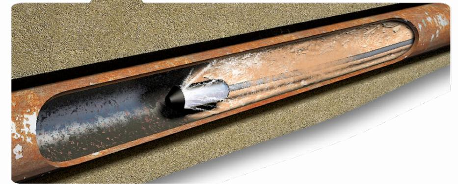
Cleaning the pipe by high pressure water flush and/or poly pig and perform inspection
